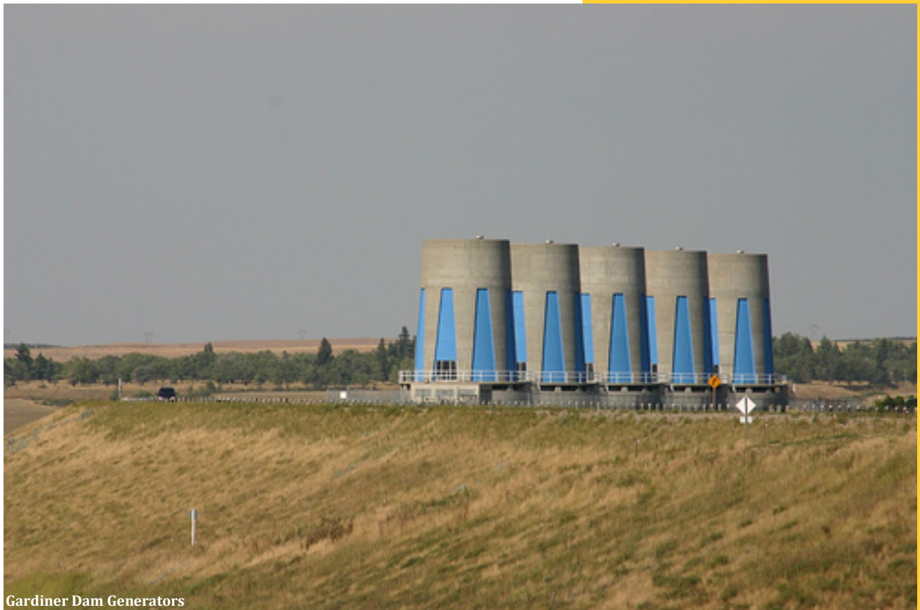
Gardiner Dam Generators
